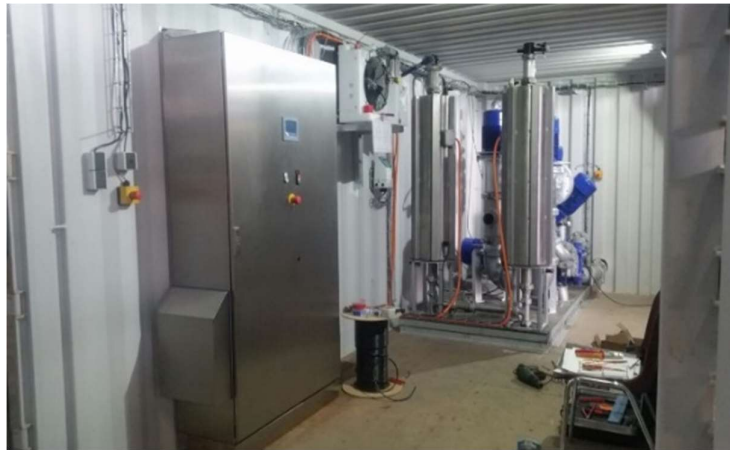
Figure 3. Example of Mobile Reactor assembly.
