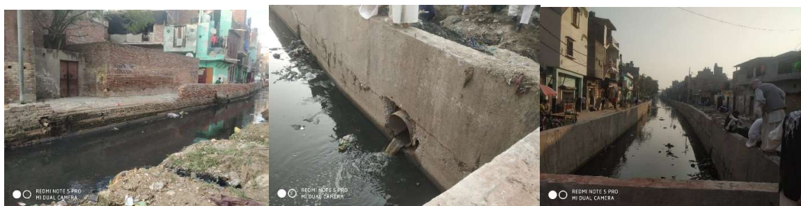
Figure 7. Untreated municipal wastewater.
