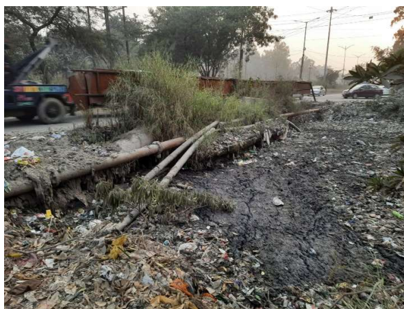
Figure 9. Crossing Electrical cables and Water pipeline
